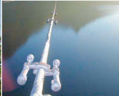
◀ Fjord crossing in Norway Sörfjorden: max. 1,600 m span length (350 kN RTS).
